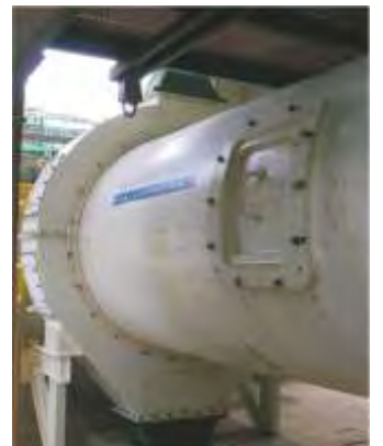
Steel Ball Mill for Calcined Clay
