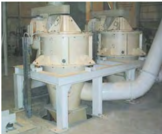
Classifying plant with 2 SCIROCCO 400SD
